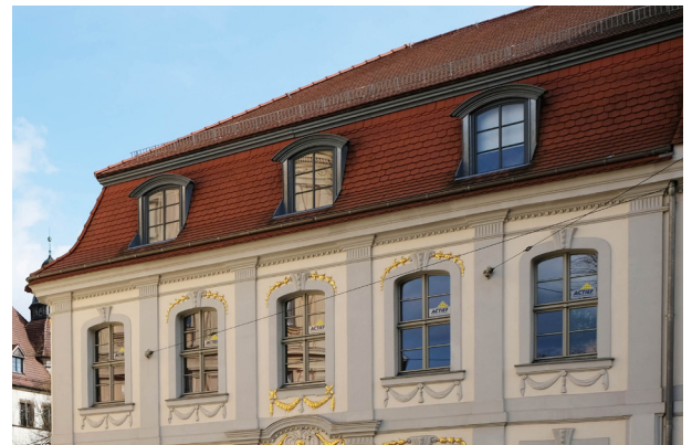
SANDOWER STRASSE Mansarddach
