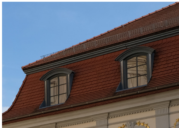
SANDOWER STRASSE Segmentbogengaupe
