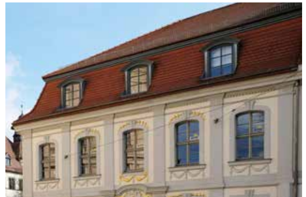
SANDOWER STRASSE Mansarddach
