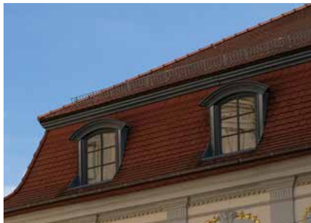
SANDOWER STRASSE Segmentbogengaupe
